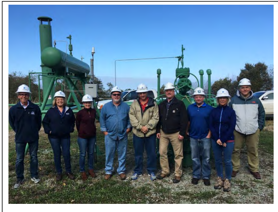
Dominion Energy North Summit Natural Gas Storage Field, Fayette County, PA
